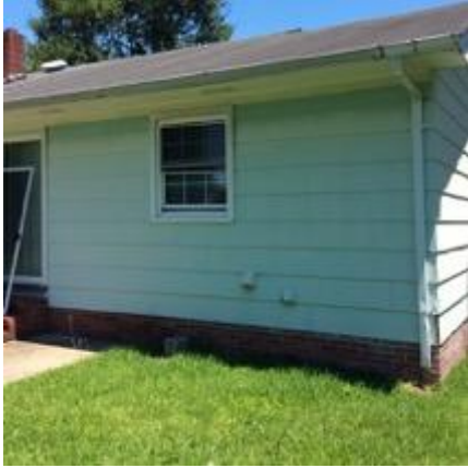
- Exterior Walls - Window was open upon arriving at home.
