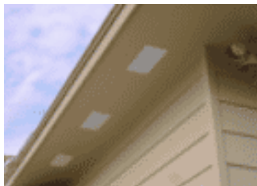
Eaves, Soffits, Fascia 2016-07-12 01:50:08
