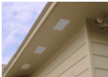
Eaves, Soffits, Fascia 2016-07-12 01:50:08
